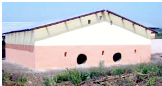
Drying house with plastic roof and heating source
